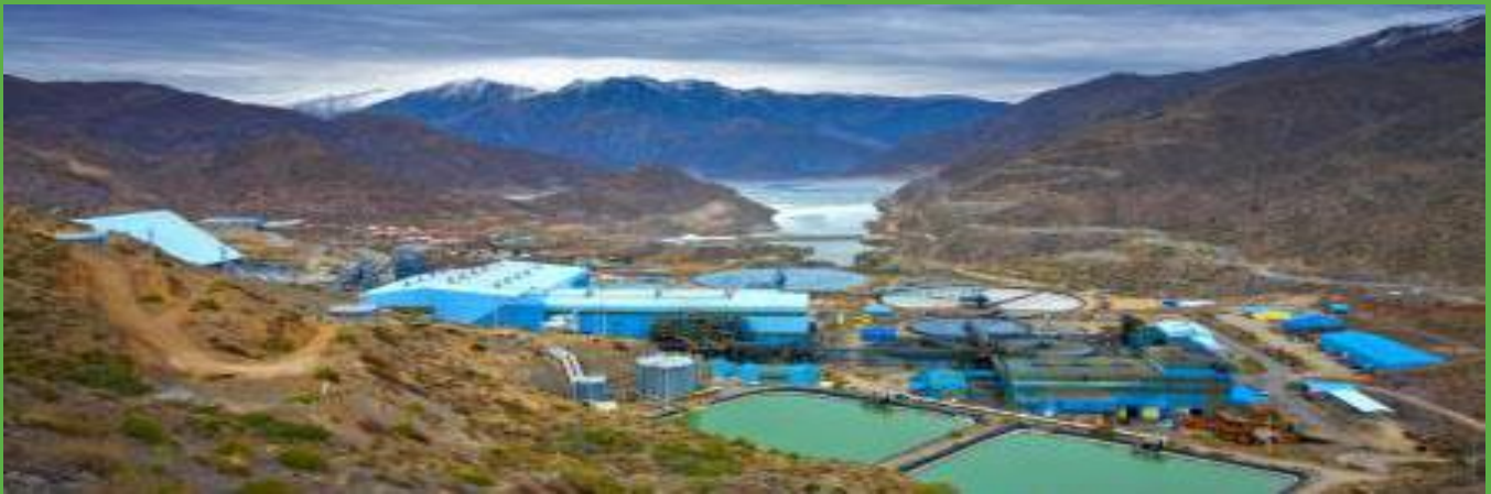
Los Pelambres Mine, panoramic view of the concentrated copper process Source: Bechtel Corporation ( www.bechtel.com/los-pelambres-mine.html )
